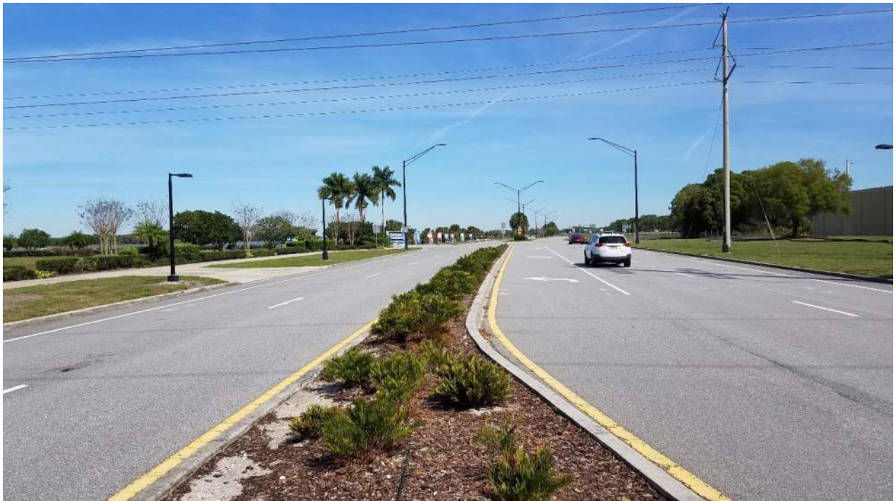
Cattlemen Road south project limit looking north
