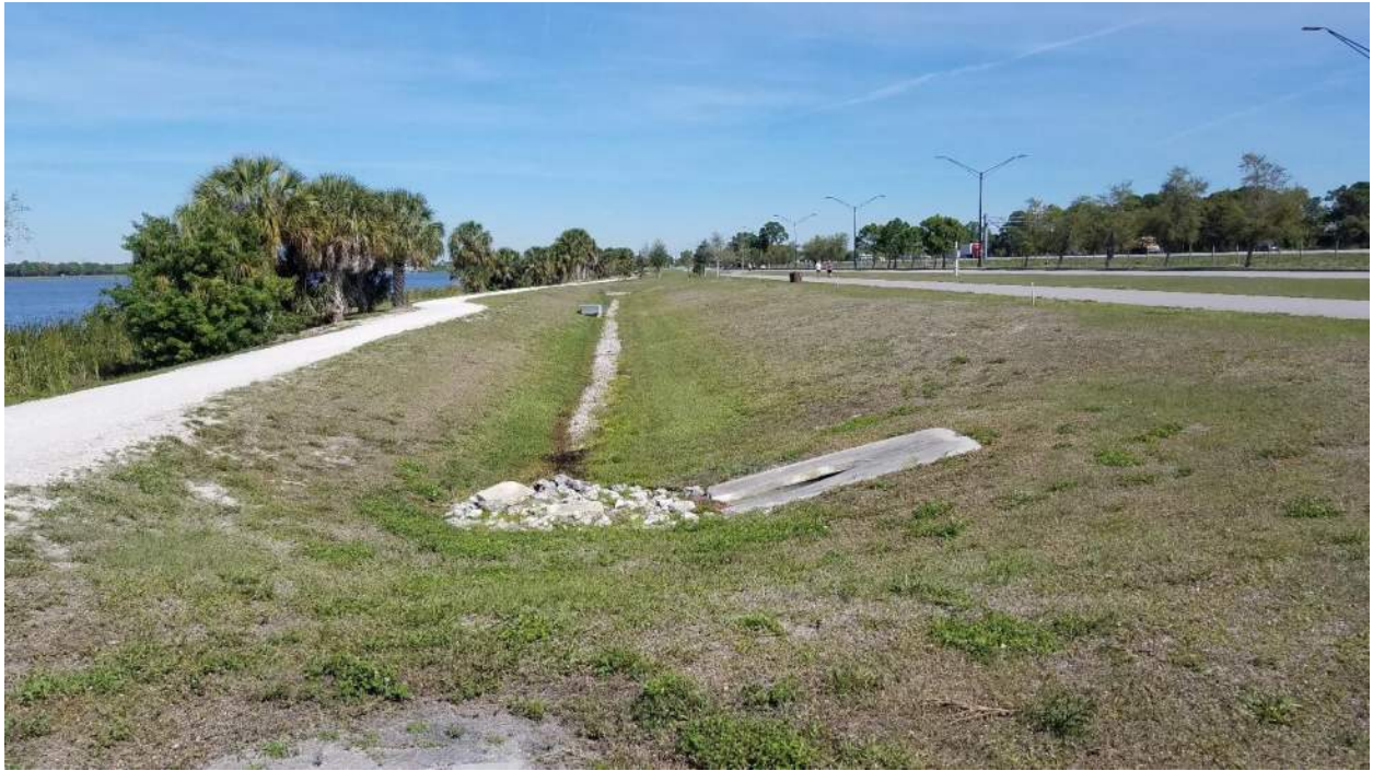
Southern area of SMF 2B looking north
