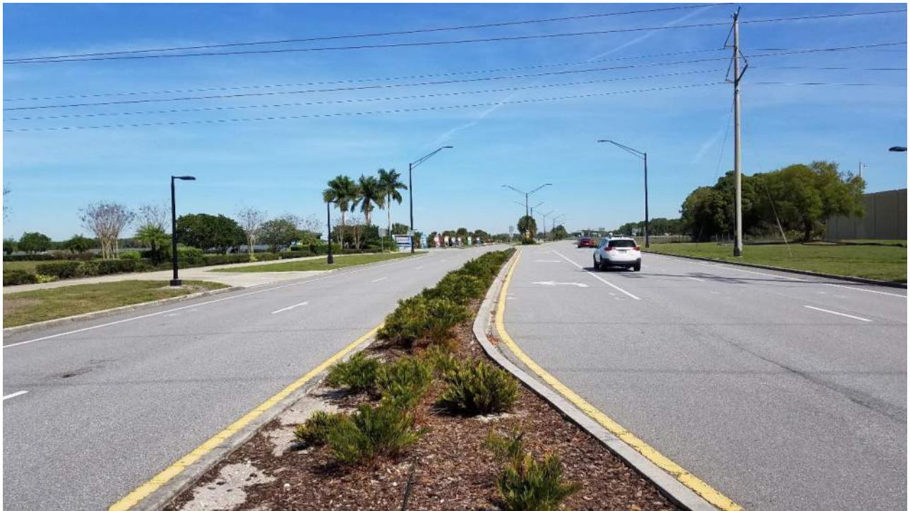
Cattlemen Road south project limit looking north
