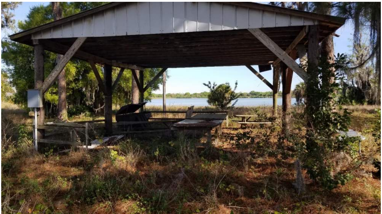
Picnic area within proposed ROW located approximately 250 feet north of the Lakewood Ranch Boulevard project limit
