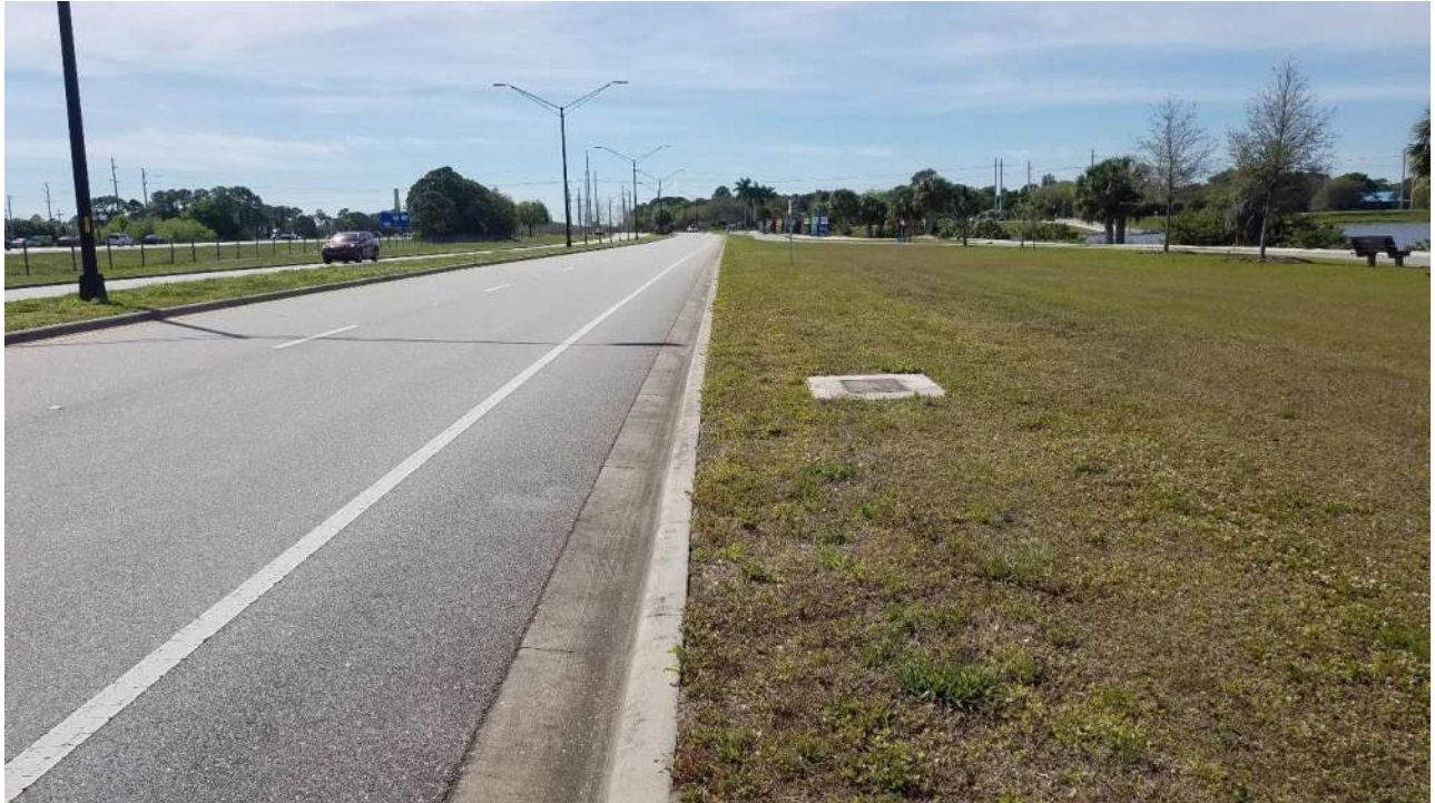
Near Cattlemen Road north project limit looking south
