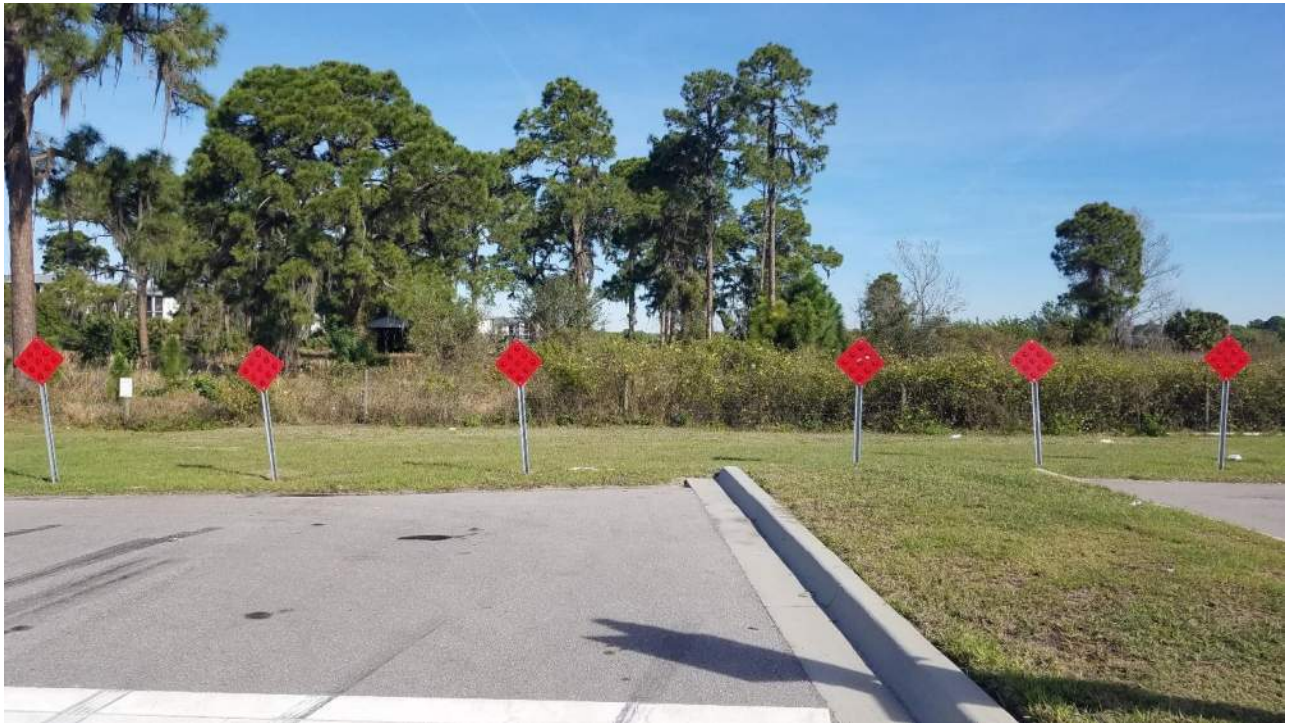
Lakewood Ranch Boulevard looking north along proposed ROW
