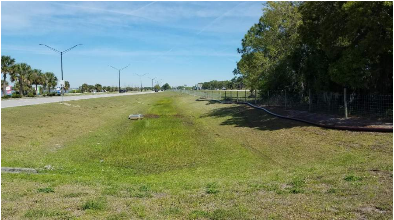
Southern area of SMF 1B looking north
